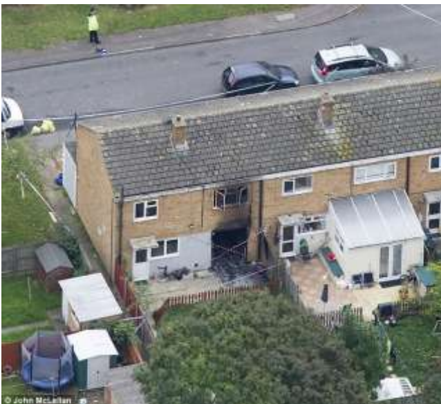
An aerial picture showing the scene at Barn Mead in Harlow after the blaze which has gutted the house
